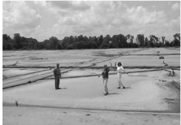
(From left) T.E. Maxson Treatment Facility Manager Pete Alfonso tours the plant’s methane gas recovery lagoon with TVA Green Power Switch officials Carmen Ledbetter and Angela Hamlin.
